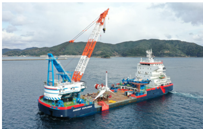
Installation of Japan's first large, commercial-scale tidal turbine in Naru Strait of Goto Islands
