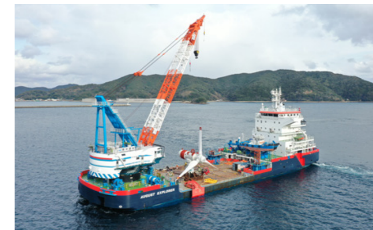
Installation of Japan's first large, commercial-scale tidal turbine in Naru Strait of Goto Islands
