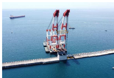
Disaster-relief work for breakwater (south) of Wakayama Shimotsu harbor north port area (1st section) (Wakayama pref.)
