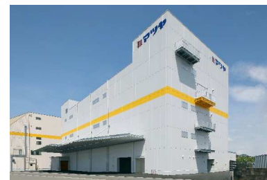
Rebuilding work for Shippo factory of Matsuya (Aichi pref.)
