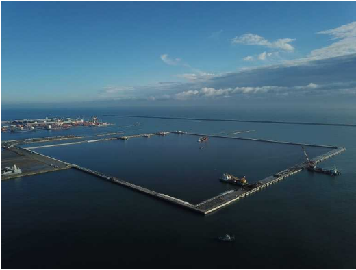
Waste materials landfill, embankment & construction work for Central pier area of Hitachi port area of Ibaraki harbor (Ibaraki)
