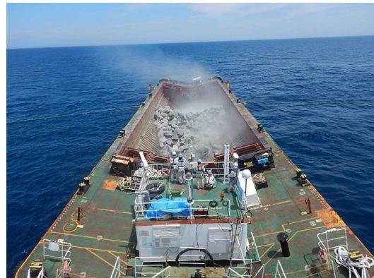
Mound bank construction work for Tsushima Strait area in 2019 (Nagasaki)
