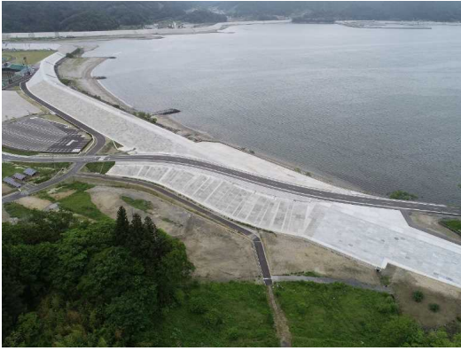
River-disaster relief work for Akamae Coast (tide embankment) (Iwate)
