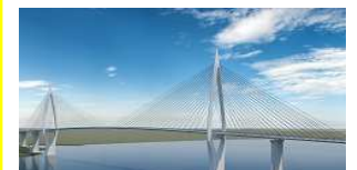
Mombasa Gate Bridge conceptional drawing (cable stayed bridge)
