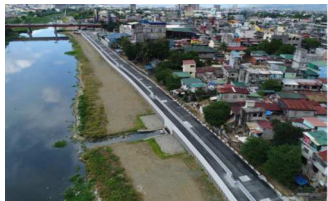
Phase III Completed (constructed by the Company)
