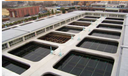
Image of water treatment plant
