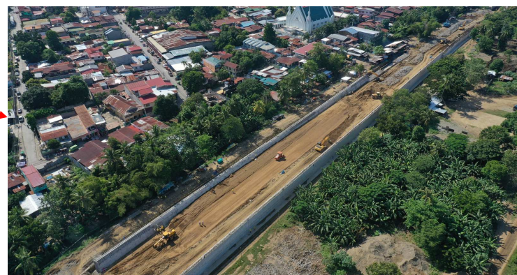
Construction status (roadbed work, subgrade work, retaining wall work)
