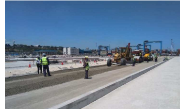
Container yard Construction status of roadbed (paving work)
