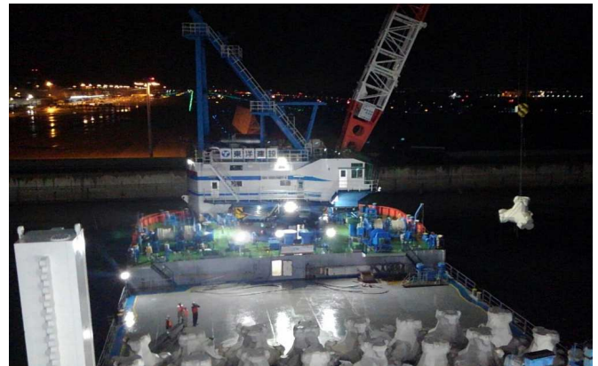
Kansai Airports Installing wave-dissipating concrete block Construction status during night-time
