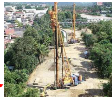
Construction status (static compaction work)
