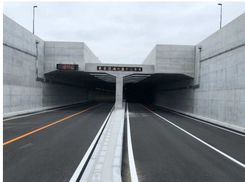
Fabrication & construction of sunken tunnel element (No.4, No.5 and No.6) for Port of Tokyo Bay Port Road Nanboku Line (Tokyo Metropolis)
