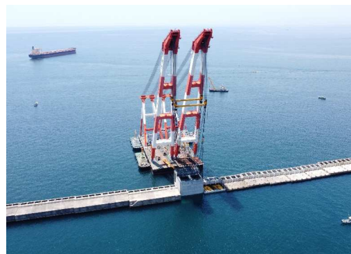
Disaster relief work for breakwater (south) of Wakayama-Shimotsu Port north port area (1st section) (Wakayama pref.)
