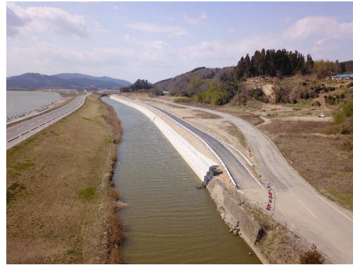
Job #: FY 2016 Prefectural bond 311 seismic disaster No. 5020-004 Disaster relief work of Osawa river (No.4) (Miyagi pref.)
