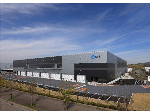
New construction for LogiSquare Kobe-West (Hyogo pref.)
