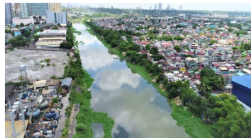
Phase IV Planned construction site
