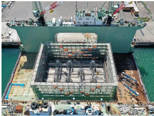
Ishikari Bay New Port Fabrication of caisson, etc. (Hokkaido pref.)
