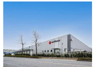
(Working title) Nishikawa Co., Ltd., New construction work of Saitama center (Saitama pref.)
