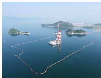
FY 2020 Yatsushiro Port & Otsuku Island, Soil improvement works for sediment disposal place (Kumamoto pref.)
