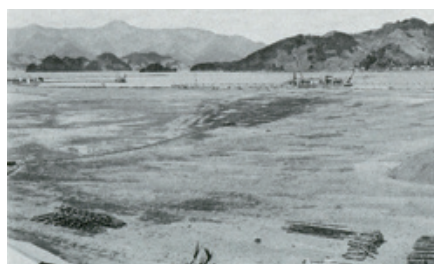
Reclamation work for Saeki naval air corps site (Oita pref.)
