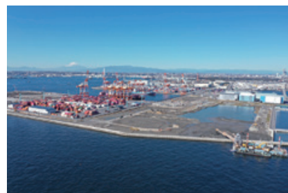
Marine transportation of landfill sediment and soil-gathering work in Minami Honmoku
