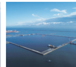
Waste materials landfill, embankment & construction work for Central pier area of Hitachinaka port area of Ibaraki harbor (Ibaraki pref.)
