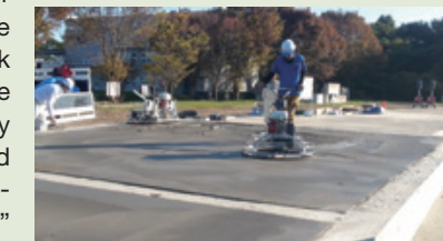
Experiment of countermeasure against cracks in floor slab (ongoing)
