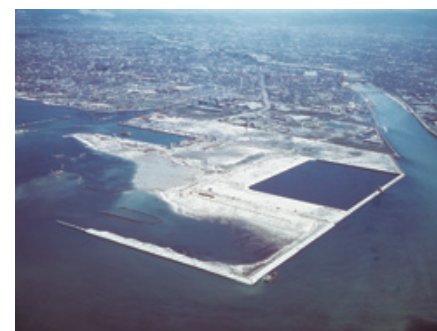
Status of Naruo Reclamation Project (April 1973)
