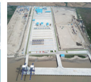
Construction of container terminal of Thilawa Port (Myanmar)
