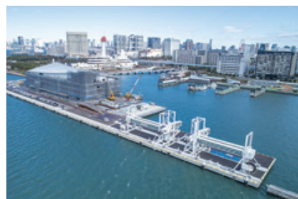
Quay construction work for the new passenger ship pier in the area No. 13
