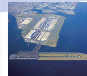
Tokyo International Airport (Haneda Airport) Runway D construction (Tokyo)
