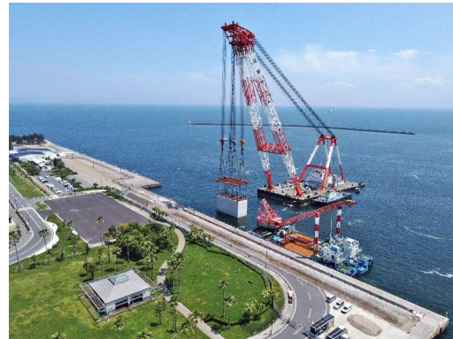
Quay construction work of Kagoshima Port (Chuoko section) in FY 2019 (Kagoshima pref.)
