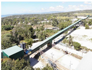
Taiheiyo Cement Corp. Construction of conveyor
