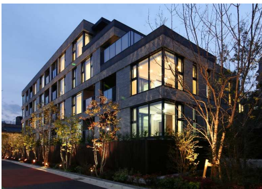
(Working title) New building construction for Sendagi 1-chome Project (Tokyo Metropolis)
