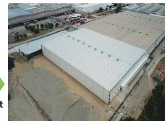
Warehouse construction for P&G (in progress)
