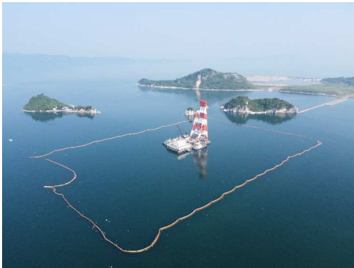
FY 2020 Yatsushiro Port & Otsuku Island, Soil improvement works for sediment disposal place (Kumamoto pref.)
