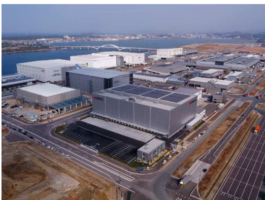
(Working title) New construction of Yokorei Island City Logistics Center (Fukuoka pref.)
