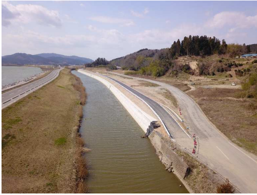
Job number: FY 2016 Prefectural bond 311 seismic disaster No. 5020-004 Disaster relief work of Osawa river (No.4) (Miyagi pref.)
