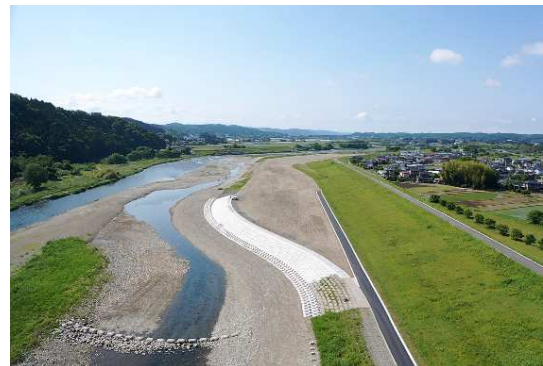
Main completed construction
