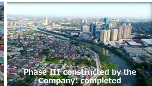
Phase III constructed by the Company: completed
