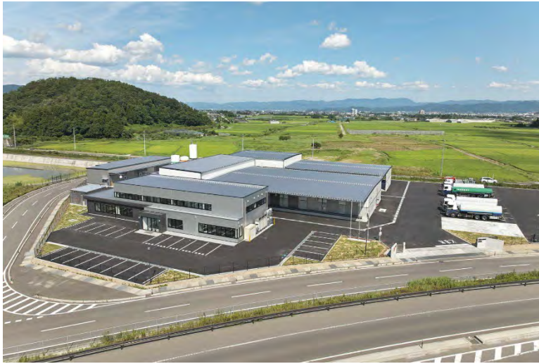
(Working title) New construction of Fukushima high pressure gas distribution center of Koatsu Gas Kogyo Co., Ltd.
