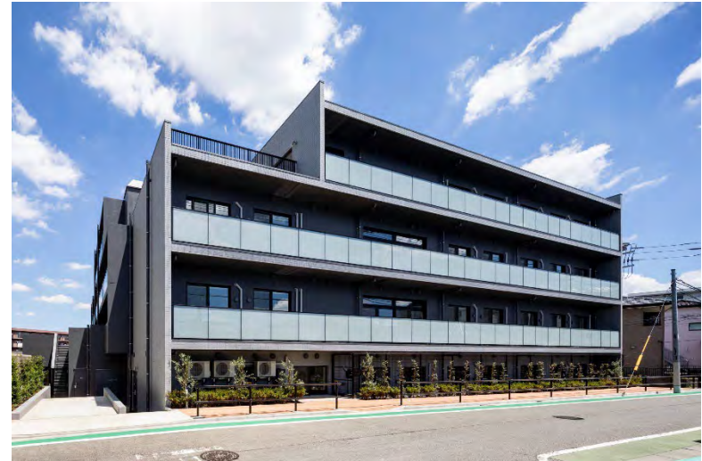
New construction work at Tokumaru 4-chome (Tokyo Metropolis)
