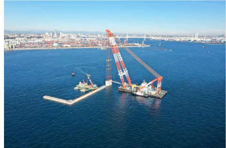
Embankment (breakwater) construction work on east side of Shin-Honmoku region of Yokohama port (Kanagawa pref.)
