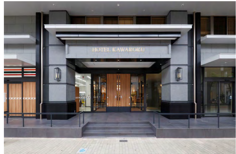
3rd term expansion and retrofitting work of Hotel Kawaroku (Kagawa pref.) 27
