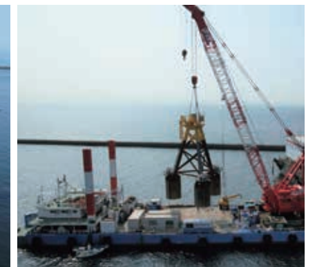
Experiment of multi buckets in a real sea area (FY 2021)
