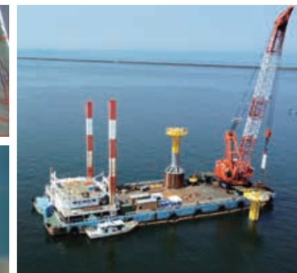
Experiment of mono bucket in a real sea area (FY 2021)
