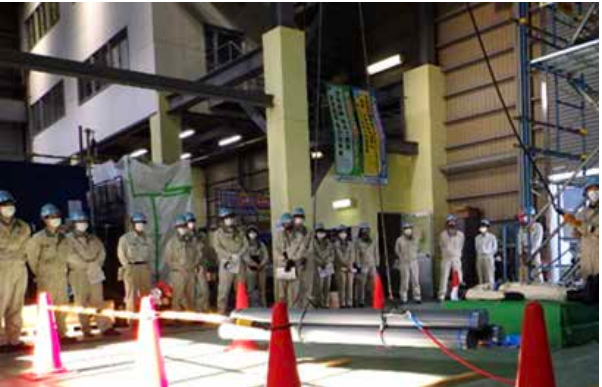
Implementation of the “3-3-3 practice” at the hoisting work “3-3-3 practice: the act of confirming the stationary state of hoisted load for 3 seconds, at 3 meters away from the hoisted load, and at 30 cm above the ground, which is aimed at maintaining the stability of the hoisted load.
