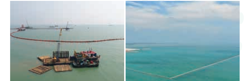
Building the foundation of the revetment by using "bamboo pile", one of the traditional Indonesian construction methods
