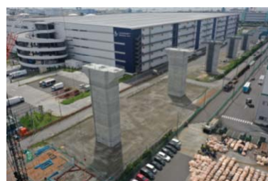
Bridge lower structure work for Higashi-Ogishima approach section of port road Higashi-Ogishima Mizue-cho Line at Port of Kawasaki (Kanagawa pref.)
