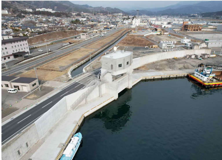
Disaster-relief for sluice gate, etc. in Kaigan-chayamae area of Ofunato Port (23 Sai - No. 166) (Iwate pref.)
