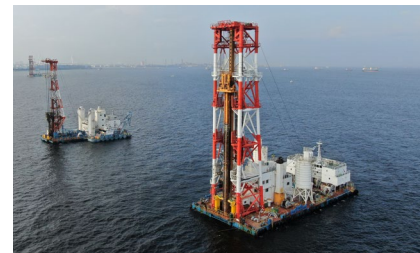
Offshore soil improvement work
