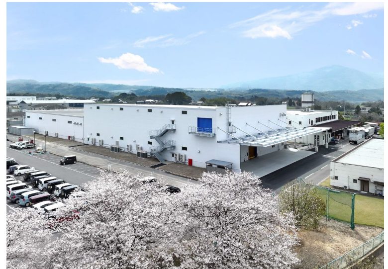
Construction work of #2 factory building of Oita Factory of Muratec Mechatronics Co., Ltd. (Oita pref.)
