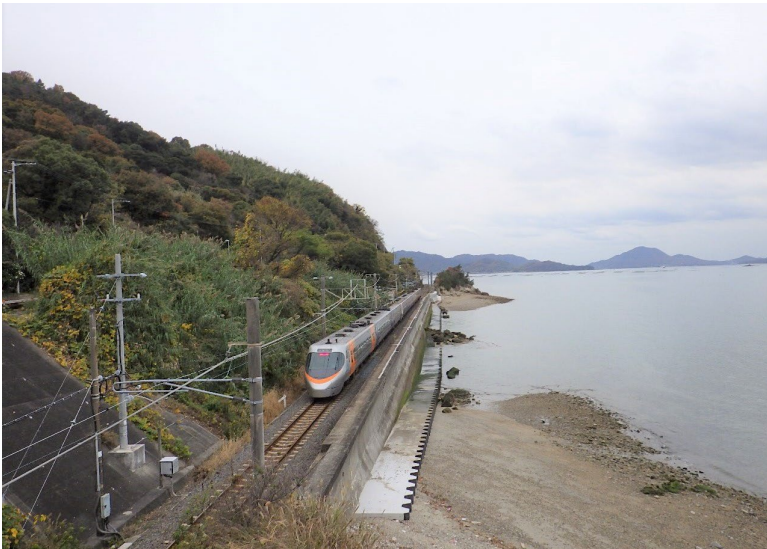
Revetment & remedial work (No.4) for Kaigan-ji & Takuma of Yosansen Line (Kagawa pref.)
