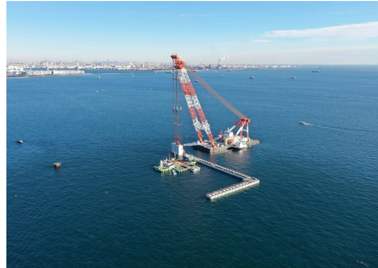
Embankment (breakwater) construction work on east side of Shin-Honmoku region of Yokohama Port (Kanagawa pref.)
