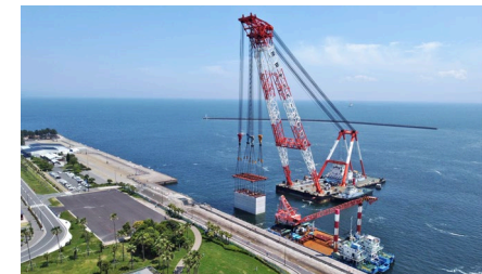
Quay wall construction
