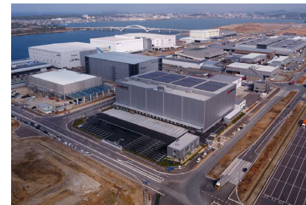
Refrigerated warehouse construction
