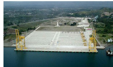
Cagayan de Oro, Philippines Container wharf construction
