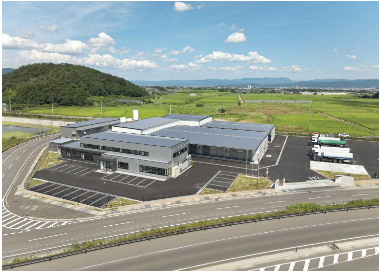
(Working title) New construction of Fukushima high pressure gas distribution center of Koatsu Gas Kogyo Co., Ltd. (Fukushima pref.)
