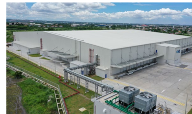
Logistics warehouse construction
