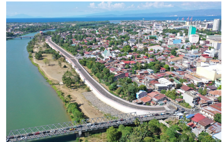
Cagayan De Oro River Channel Improvement
