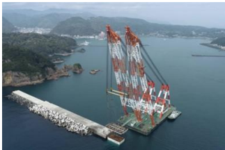
Caisson Installation Using Japan’s Largest Crane Vessel at Shimoda Port Breakwater (West) E District Construction Project in FY2023
