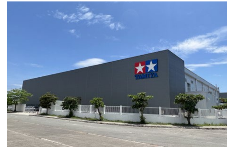
TAMIYA Philippines, Inc. New Factory Building
