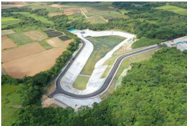
Ishigaki (5) Construction Work (2)
