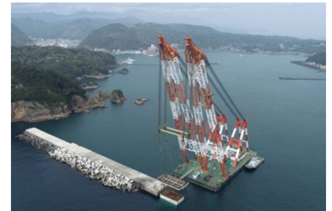
Caisson Installation Using Japan's Largest Crane Vessel at Shimoda Port Breakwater (West) E District Construction Project in FY2023
