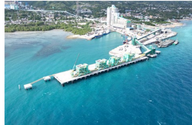
SEDC NEW JETTY, DOLPHINS AND ECHO BEACH PLATFORM PROJECT
