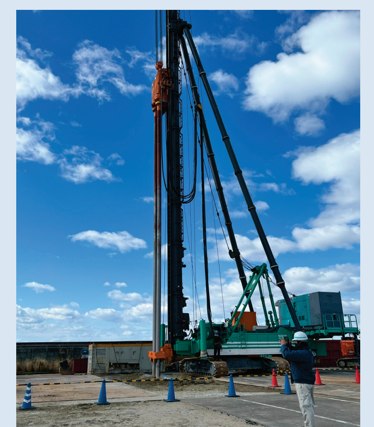
Ground Improvement Using the CDM Method
