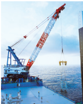
隠岐島沖で魚礁の据付を行うAUGUST EXPLORER
