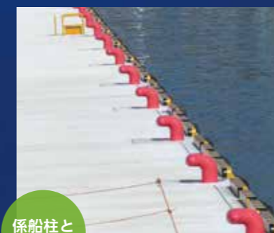
係船柱と車止め
