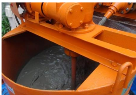
(a)基材練混ぜ状況
