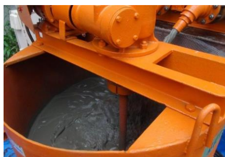
(a)基材練混ぜ状況
